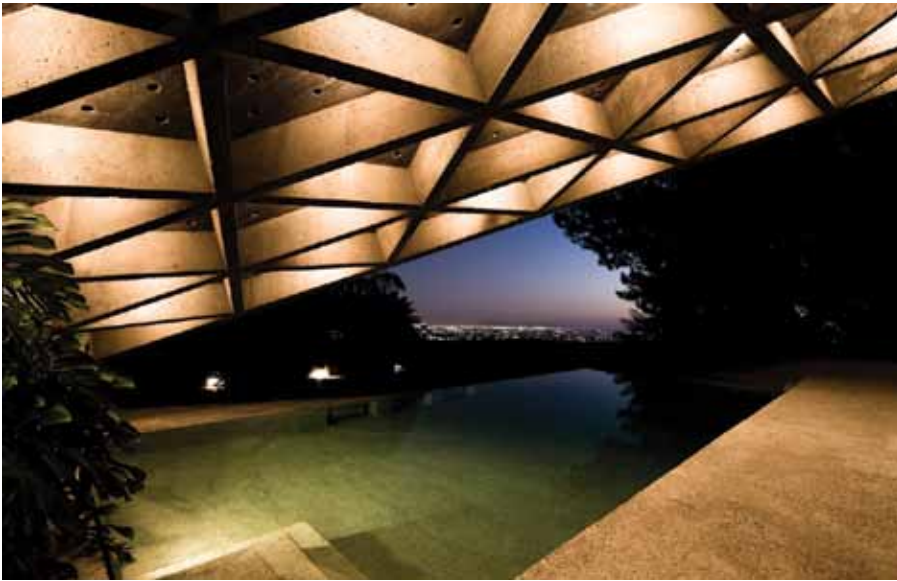
Above: A coffered roof shades part of the terrace and pool at the Sheats-Goldstein residence. Below: The Garcia house demonstrates Lautner's ability to mold concrete into unconventional forms. Both images courtesy of Francois Dischinger.
